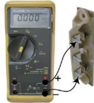
Transformer Secondary Circuit
